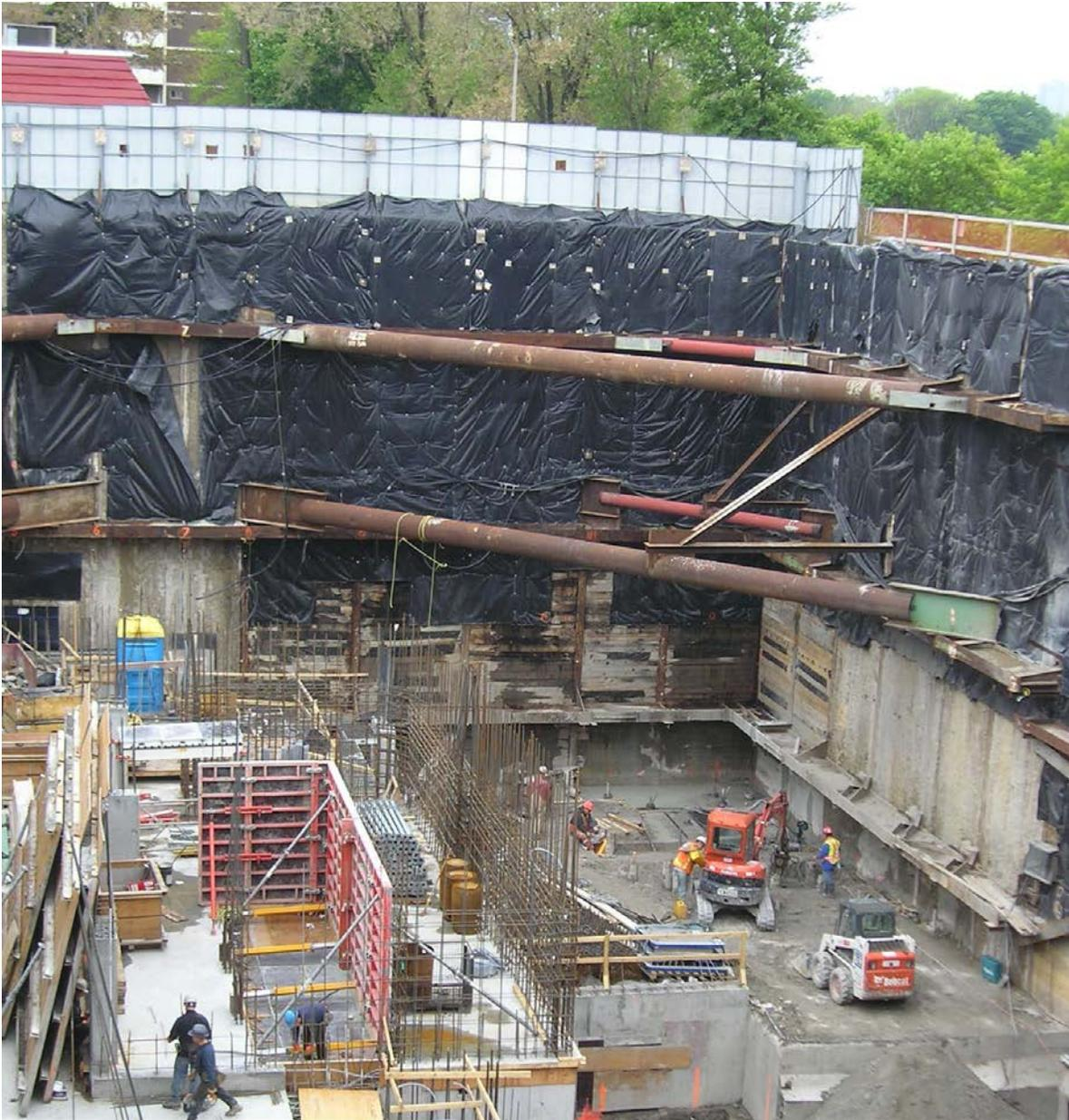
FIG. 2: View of the southwest corner of the Skyy project – note the large corner brace at 6 m above grade
