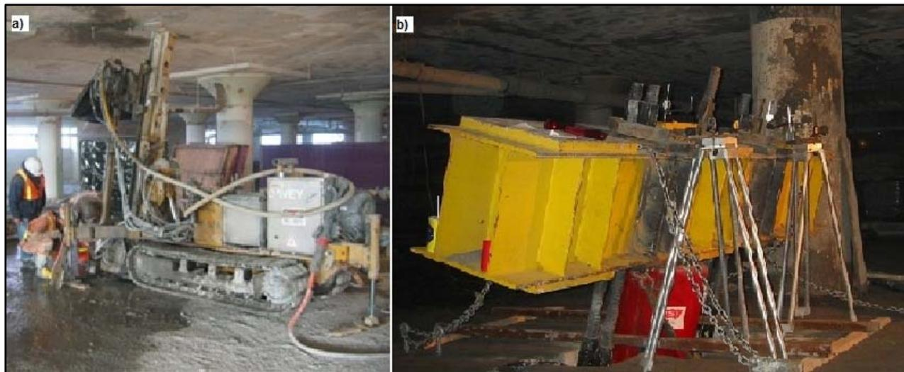
Figure 1. a) Low-head room drilling inside the existing basement at Tip Top Lofts; b) Micropile load test arrangement
